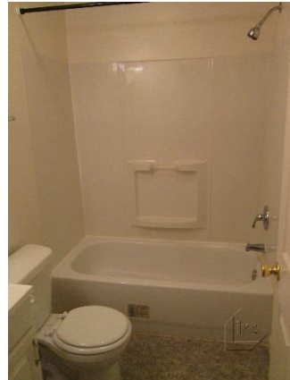
Unit A Bathroom (Photo Taken on May 2, 2016)
