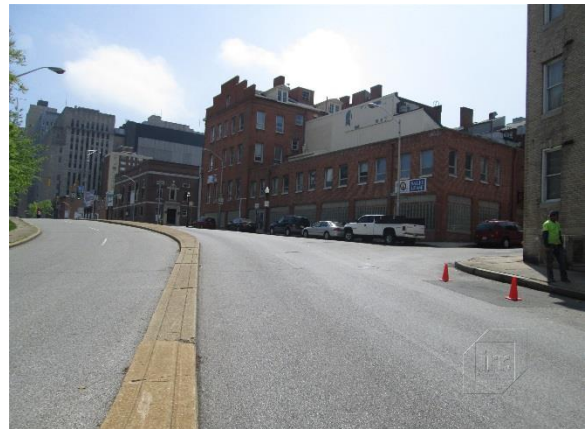
Saint Paul Place Looking Southwest (Photo Taken on May 2, 2016)
